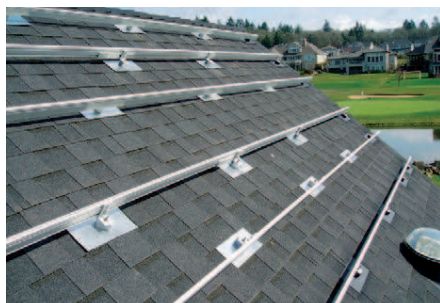
SHINGLE ROOF MOUNTING STRUCTURE FOR PITCHED ROOF
